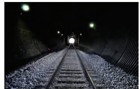
Type III optics on our Champ VMV LED minimize light spillover onto the walls and direct light to the ground where it's needed
